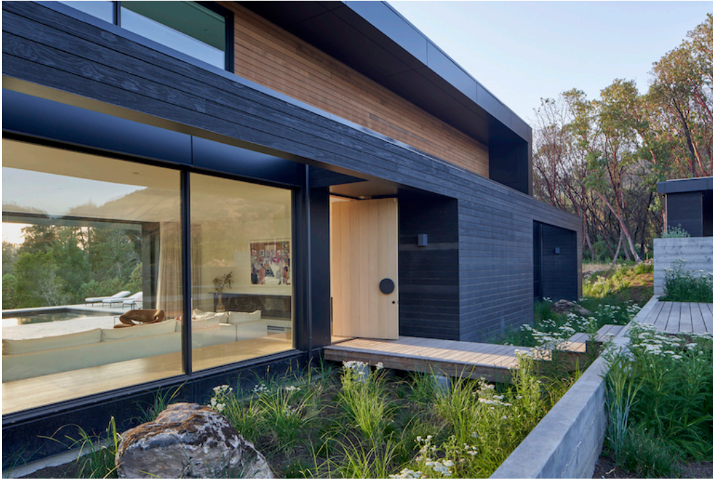
The exterior of this home is mostly metal framing and shou sugi ban, a Japanese charred treatment that's resistant to fire. Photo by Bruce Damonte.
